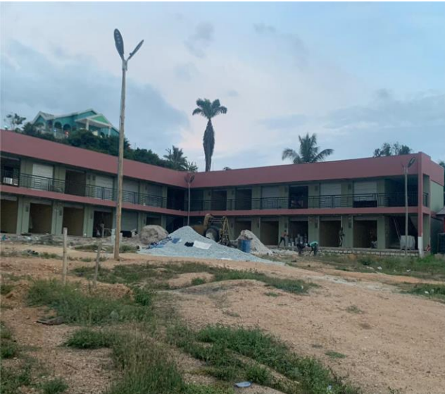
Construction of 60 No. lockable stores at Anomabo
