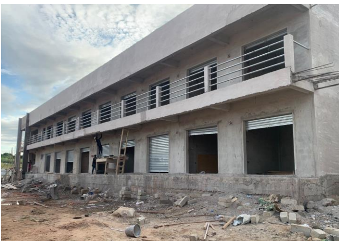
Two (2) Storey Thirty-Six (36) No. Lockable Stores at Mankessim-Lot 1
