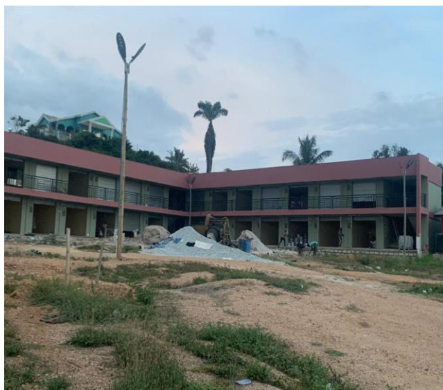
Construction of 60 No. lockable stores at Anomabo
