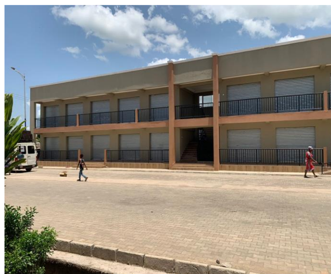
20 Lockable Stores at the Ansa Park, Mankessim (UDG 3)
